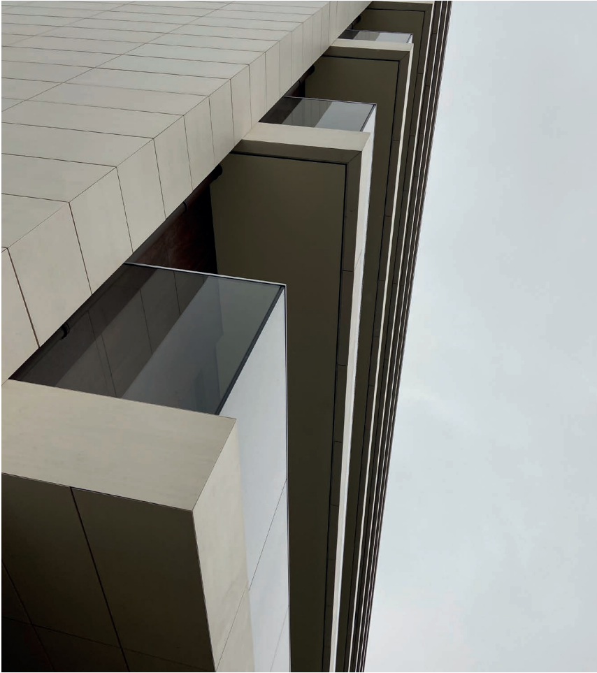
PORTUGAL - GAIA FLATS RESIDENTIAL BUILDING
